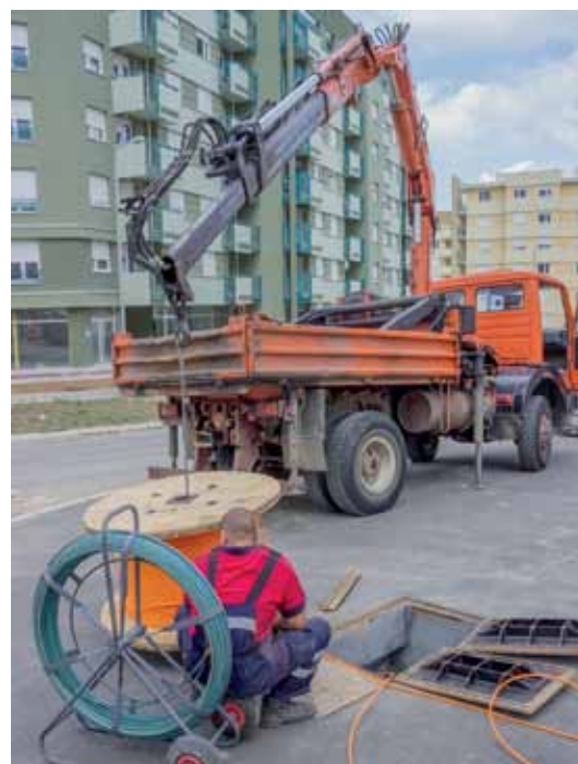
Deploying FTTH in urban areas presents construction challenges
